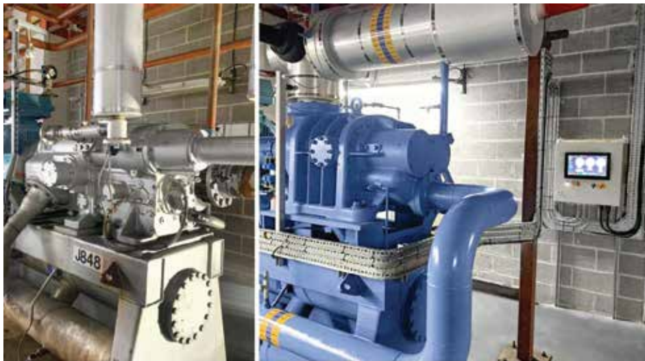
A GEA compressor replacement gives new life and increased efficiency to this existing screw compressor package by another manufacturer, as illustrated by this before & after example. A GEA Omni control panel retrofit is also part of this equipment upgrade.
